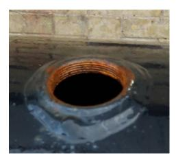
Insert the 2" to 1" NPT adapter. Ensure that it is rightly sealed and watertight - e.g. PTFE tape around the threads can help ensure a good seal.
